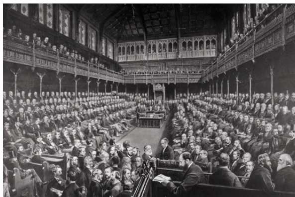
Chamber of the House of Commons, 1875
